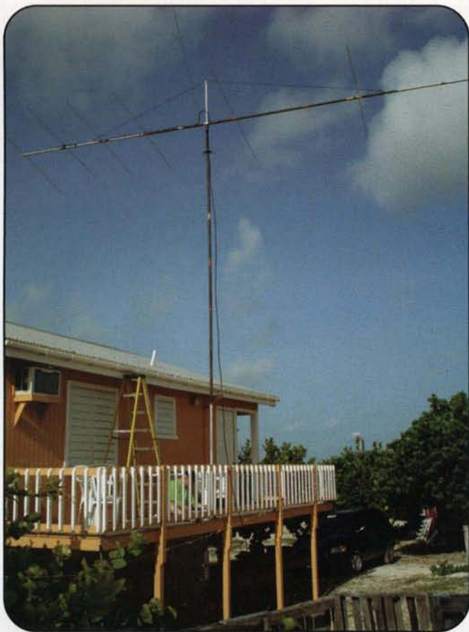
The 24-foot rotating mast, elements, and boom for the 7-element Yagi.
