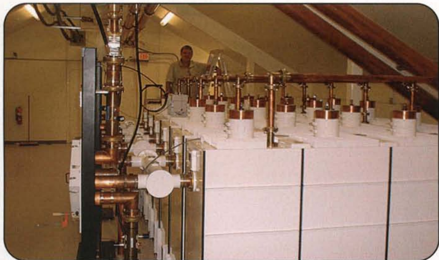
Photo 5. These filters combine five transmitters onto one antenna. Three of the transmitters go out right-hand circular polarized and two of the transmitters go out left-hand circular polarized.
